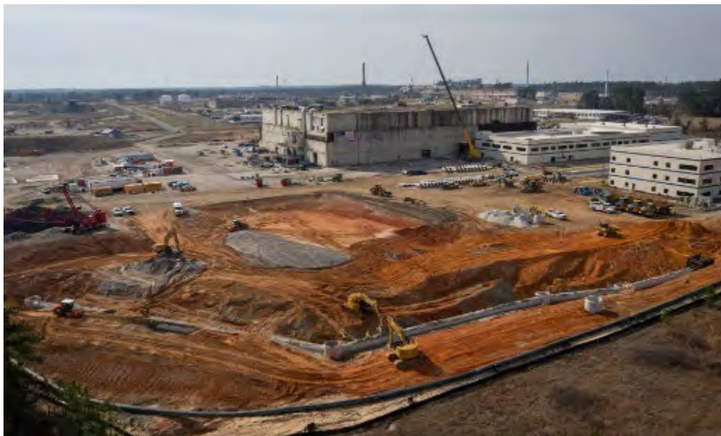
Figure 3. An aerial photograph of excavators and other heavy equipment conducting site preparation work next to the existing structures, which includes sand filter excavation.
