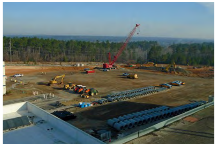
Figure 44. Photographs showing before (left) and after (right) the removal of a parking lot and the start of sand filter excavation. These photographs were taken from the existing structure for the Savannah River Plutonium Processing Facility project.
