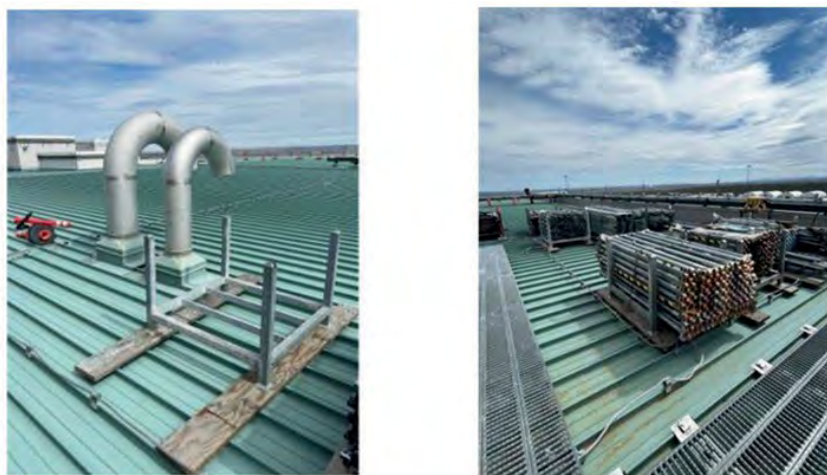
Figure 57. Discharge pipes (left) and metal scaffold pipe (right) located above air terminals.
