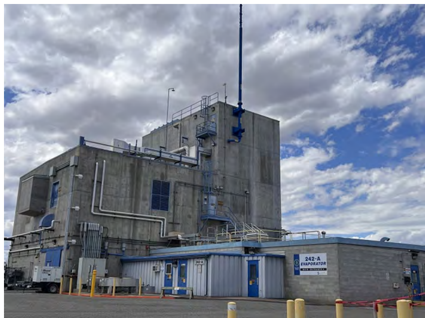
Figure 18. Hanford 242-A evaporator exterior.
