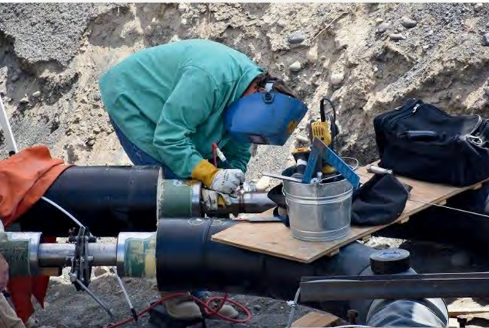
Figure 16. Worker installing a transfer line that will transport waste between facilities at Hanford site.
