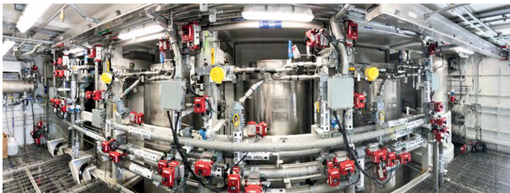
Figure 20. Tank side cesium removal system process enclosure.
