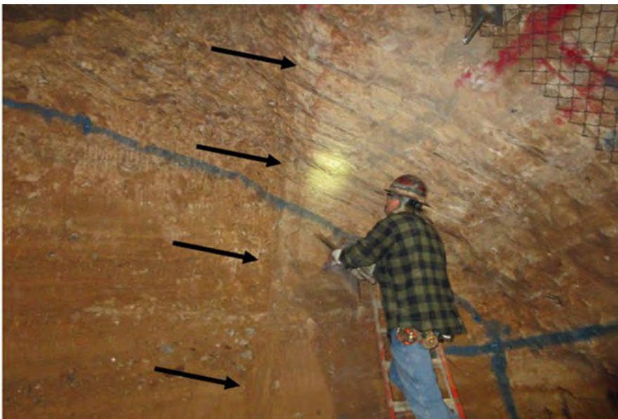
Figure 39. Arrows pointing to the fault plane, showing evidence of historic seismic activity of the faults present within PULSE.
