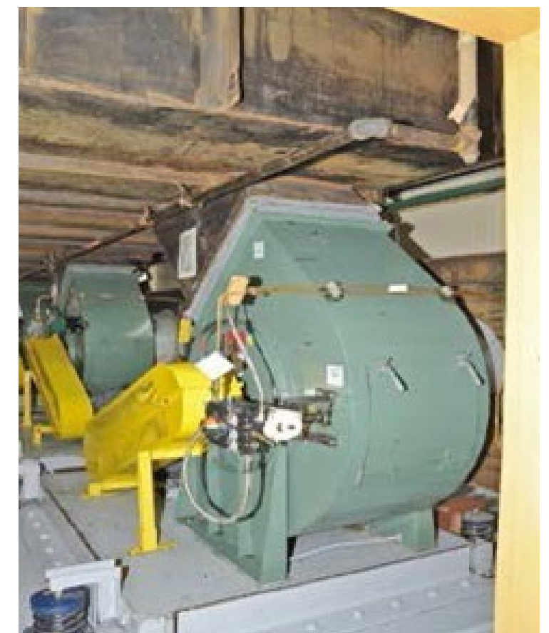
Ventilation system fan planned for replacement.
