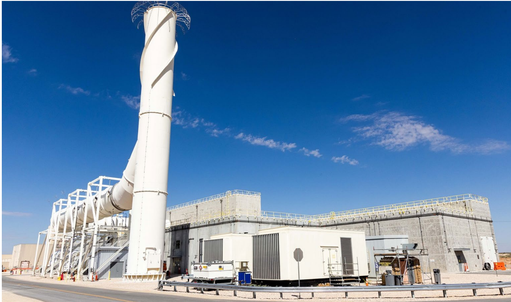
Safety Significant Confinement Ventilation System
