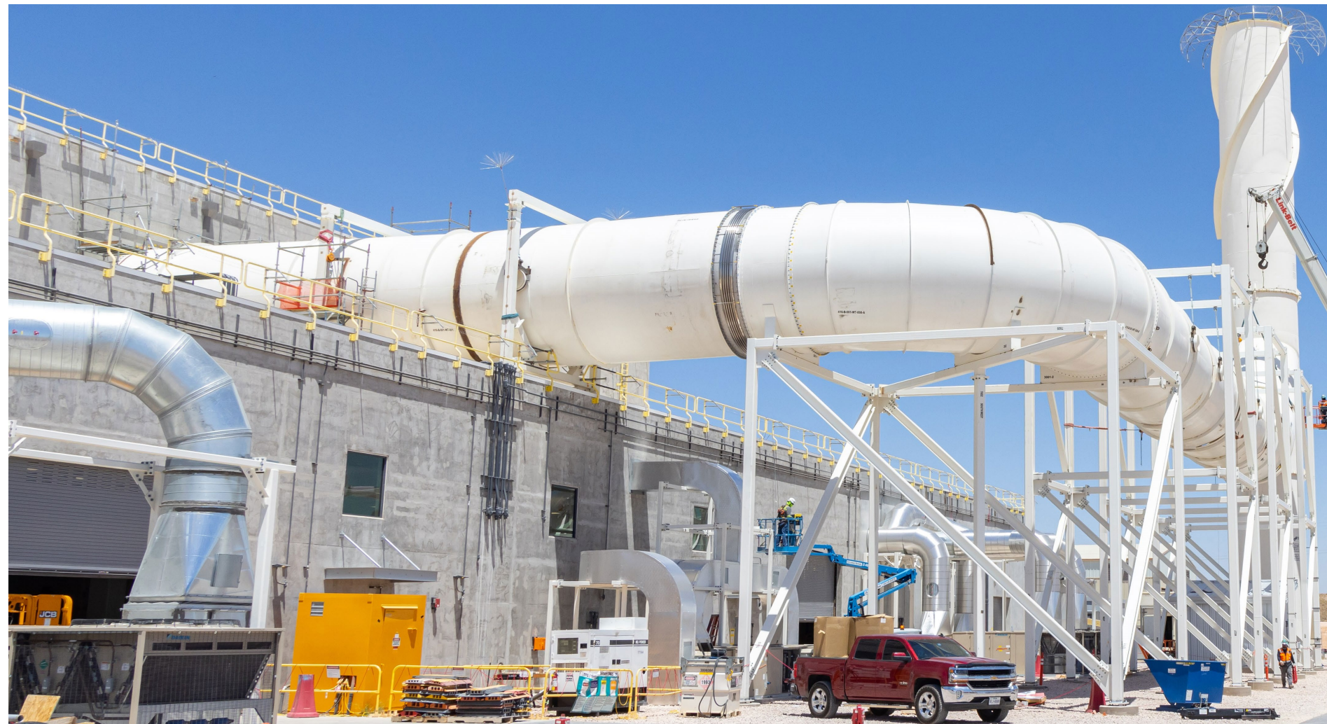
Safety Significant Confinement Ventilation System
