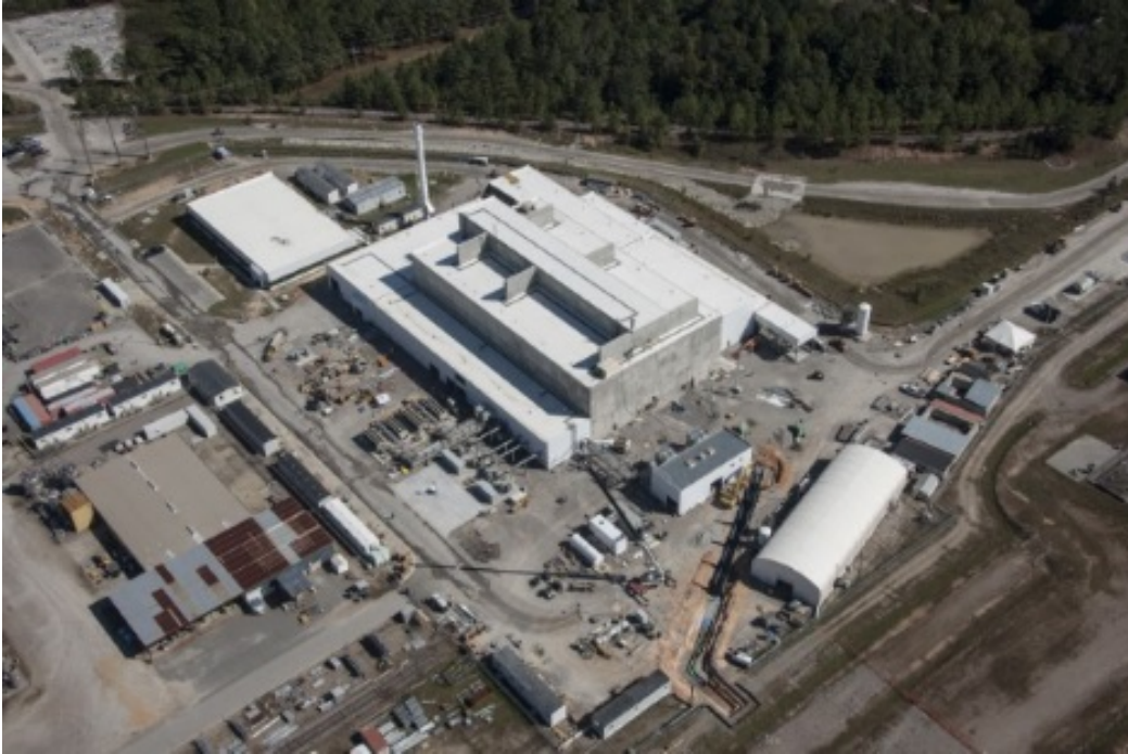
Salt Waste Processing Facility, Savannah River Site
