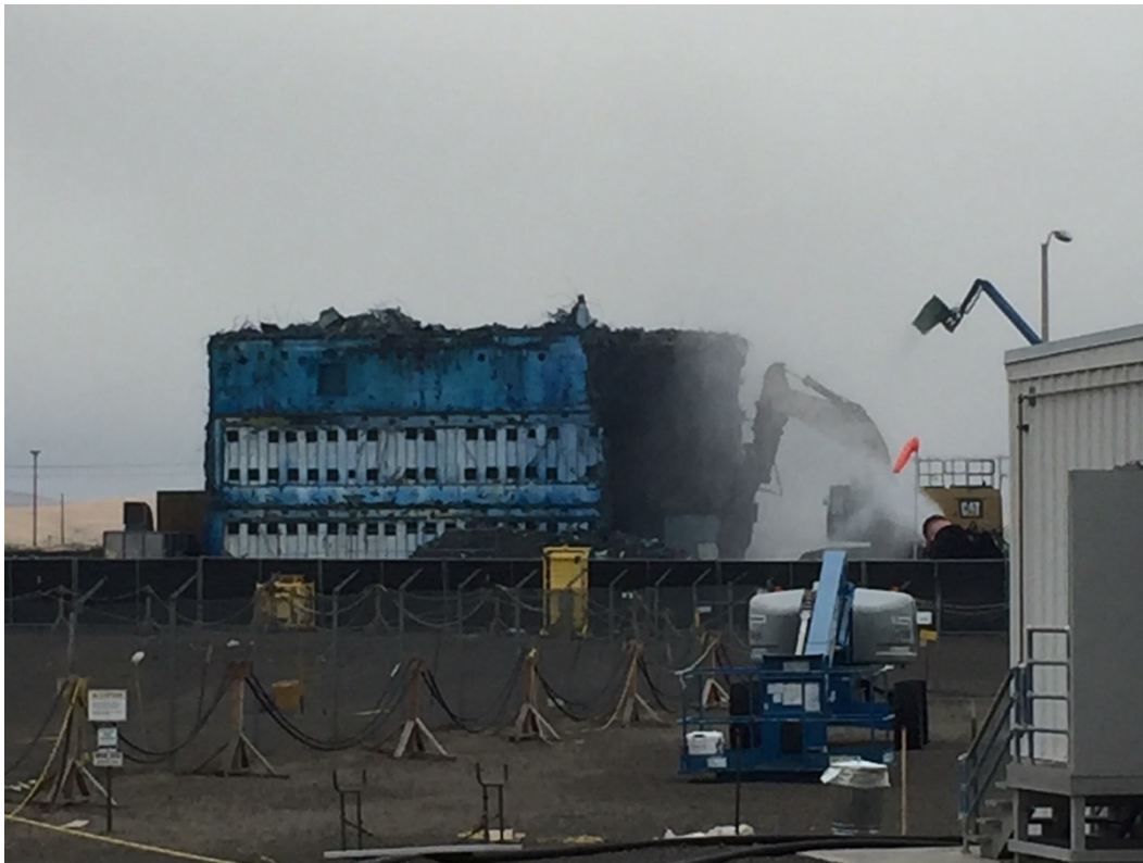
Demolition of the Hanford Plutonium Finishing Plant
