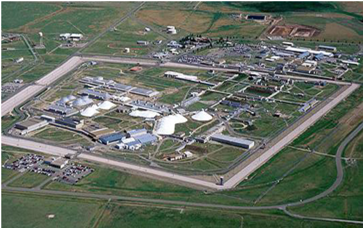
Nuclear Explosive Facilities at the Pantex Plant
