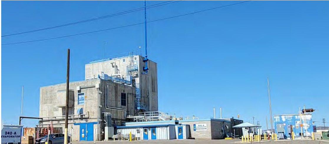
Figure 11. 242-A Evaporator Facility at Hanford Site
