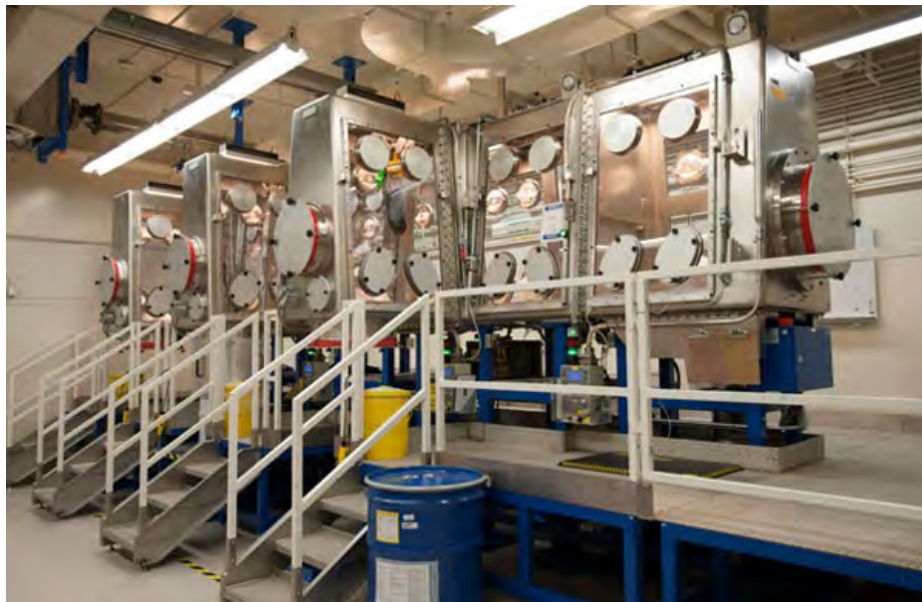
Figure 18. Centralized Waste Processing Line gloveboxes in the Plutonium Facility.
