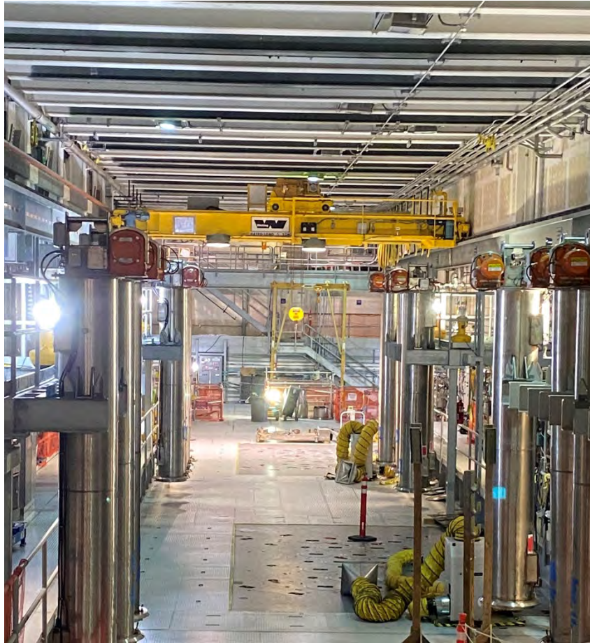
Figure 19. Melter gallery in the Low-Activity Waste facility.
