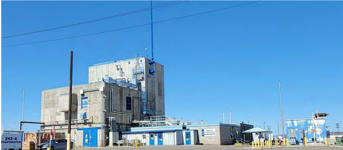
Figure 11. 242-A Evaporator Facility at Hanford Site
