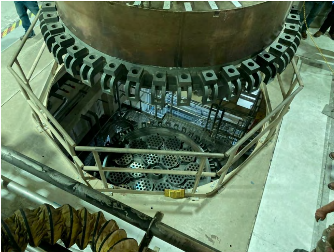
Figure 16. Opening the process gas filter on the Integrated Waste Treatment Unit at INL.
