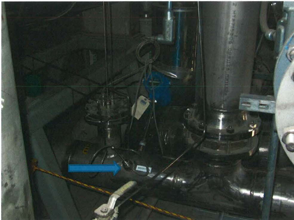
Figure 4: AZ-102 Flow Test Ports
