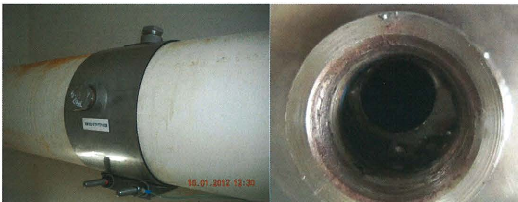
Figure 2: Typical Flow Test Port
