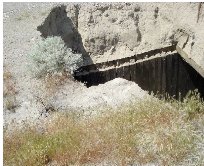
Hanford PUREX Tunnel, May 2017
